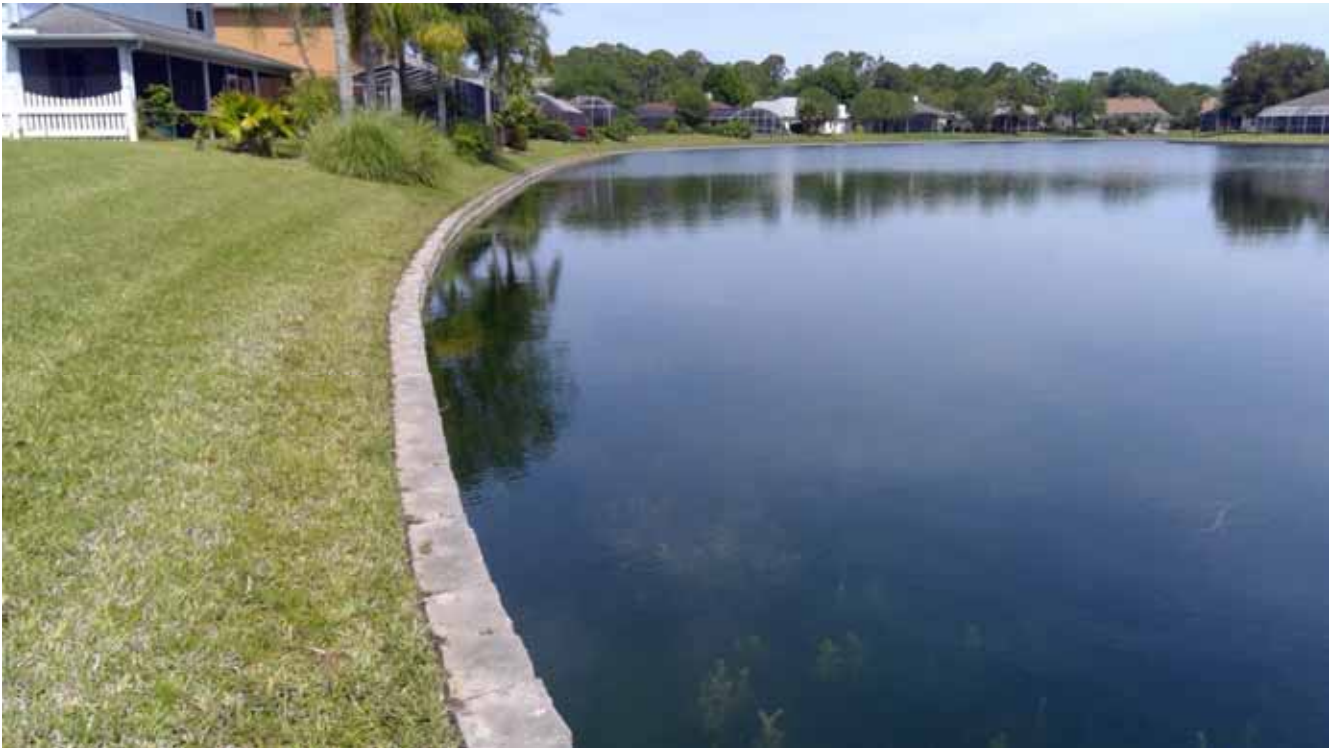
Bulkhead - Linkside Lake
