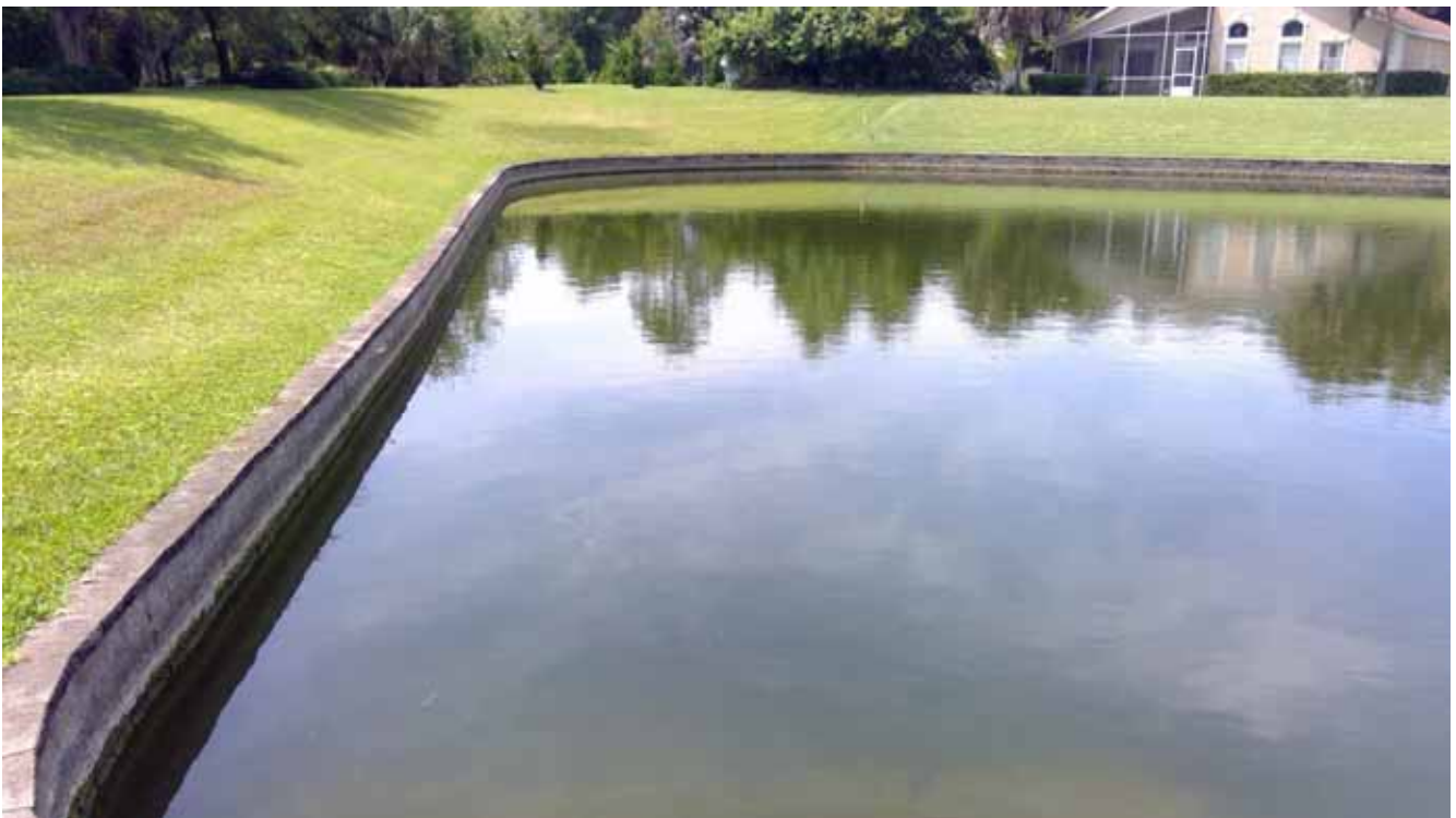
Bulkhead - Lake Haven
