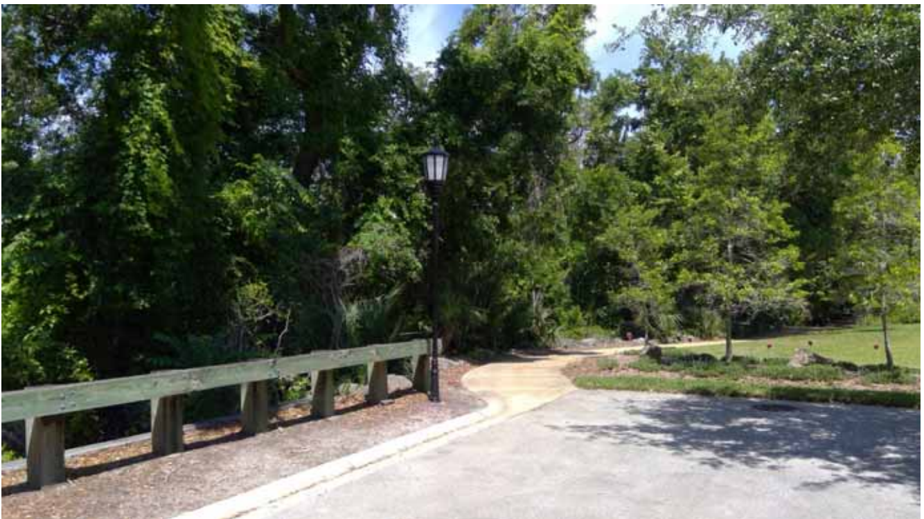
Lighting - Esplanade Walkway
