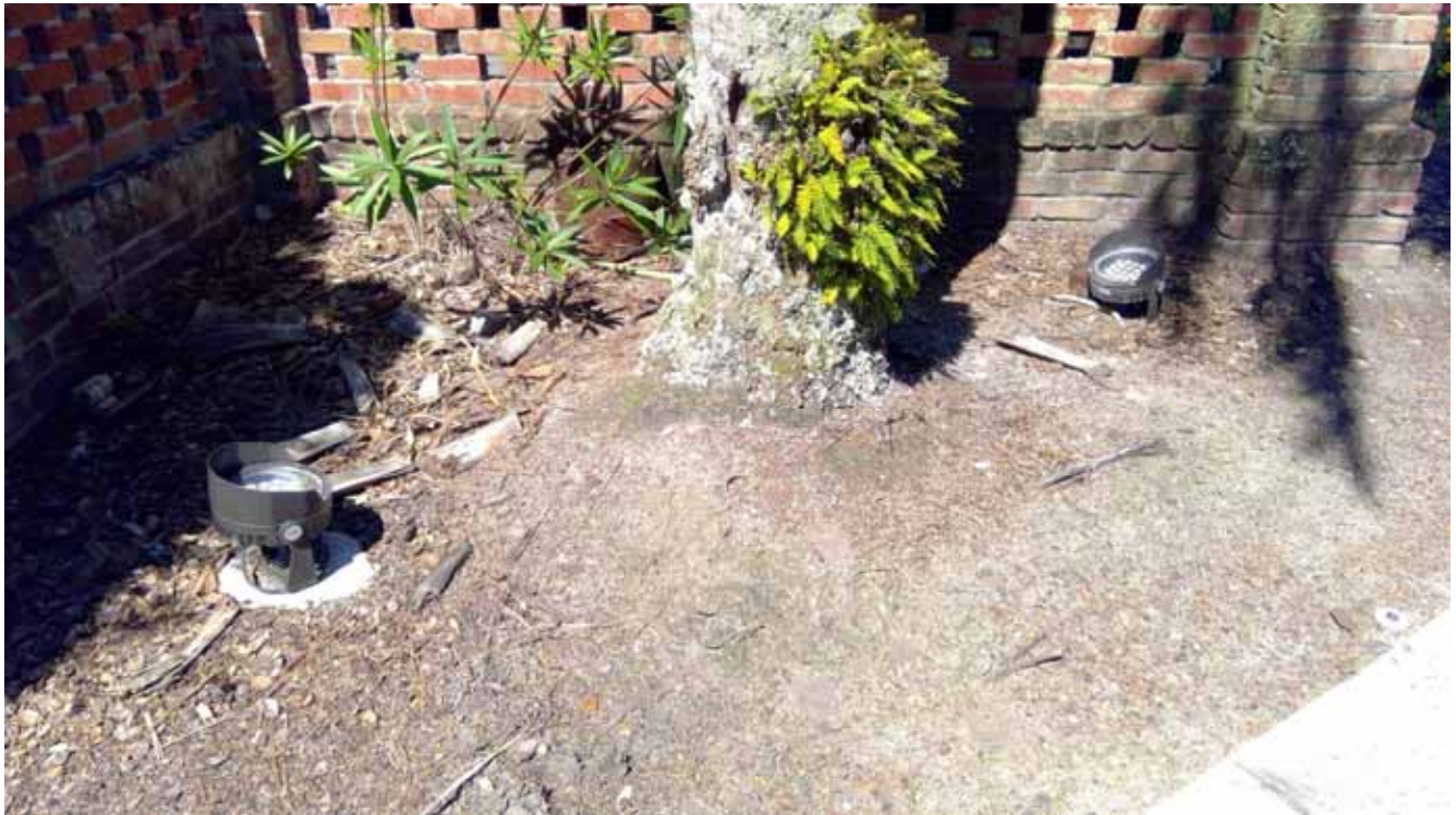
Entry Lighting - The Crossings
