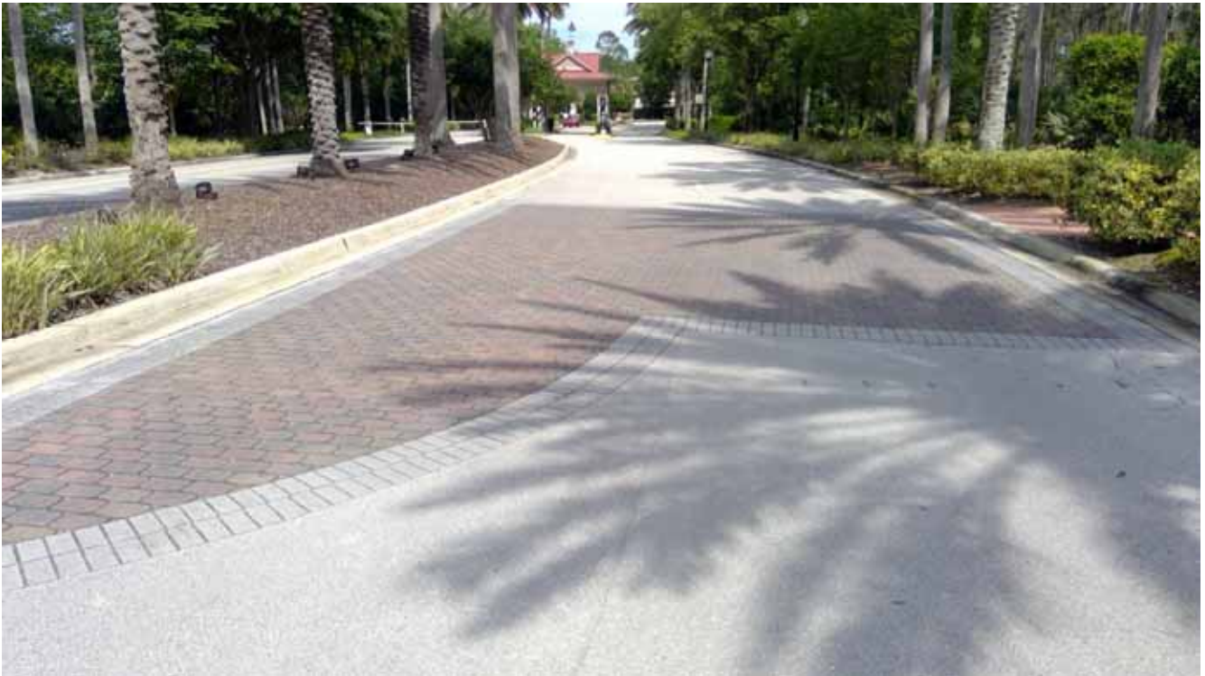
Pavers - South Entry
