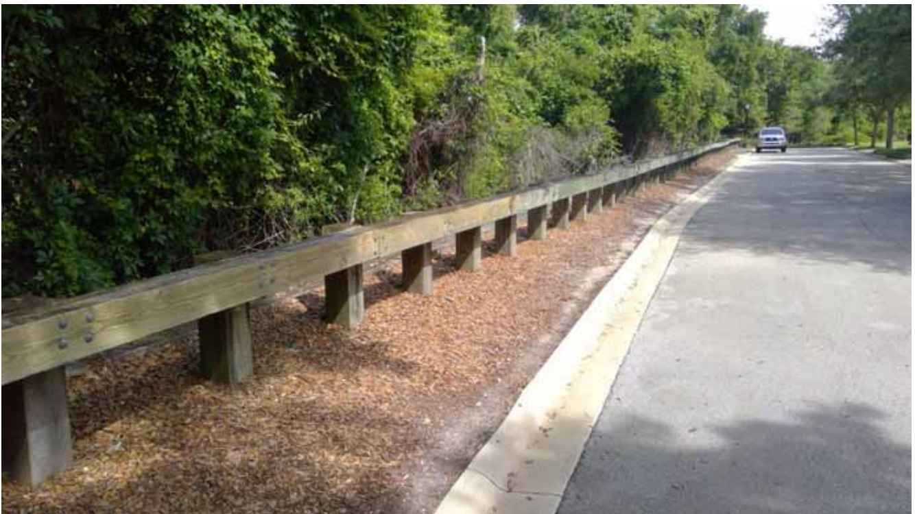
Guard Rail - River Trail Drive
