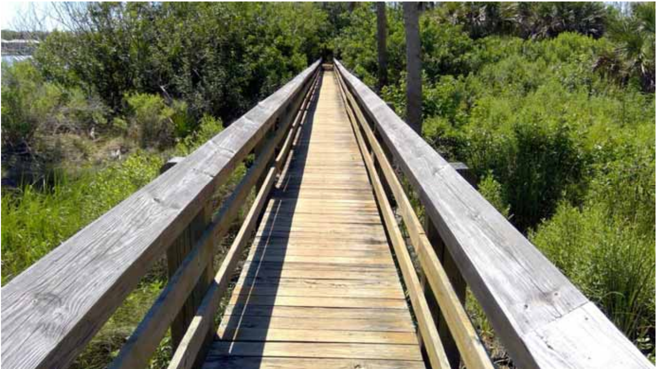
Boardwalk - The River Club
