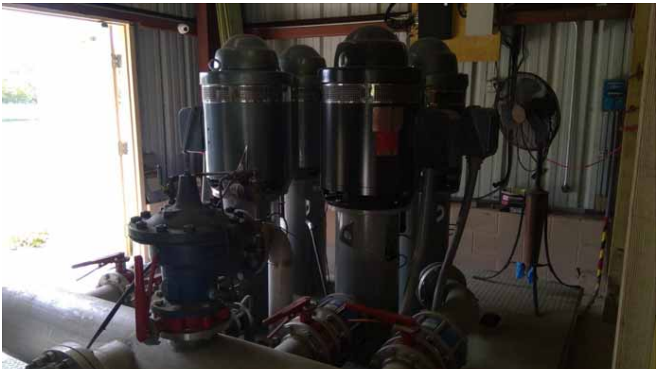
Irrigation Pump/Motor
