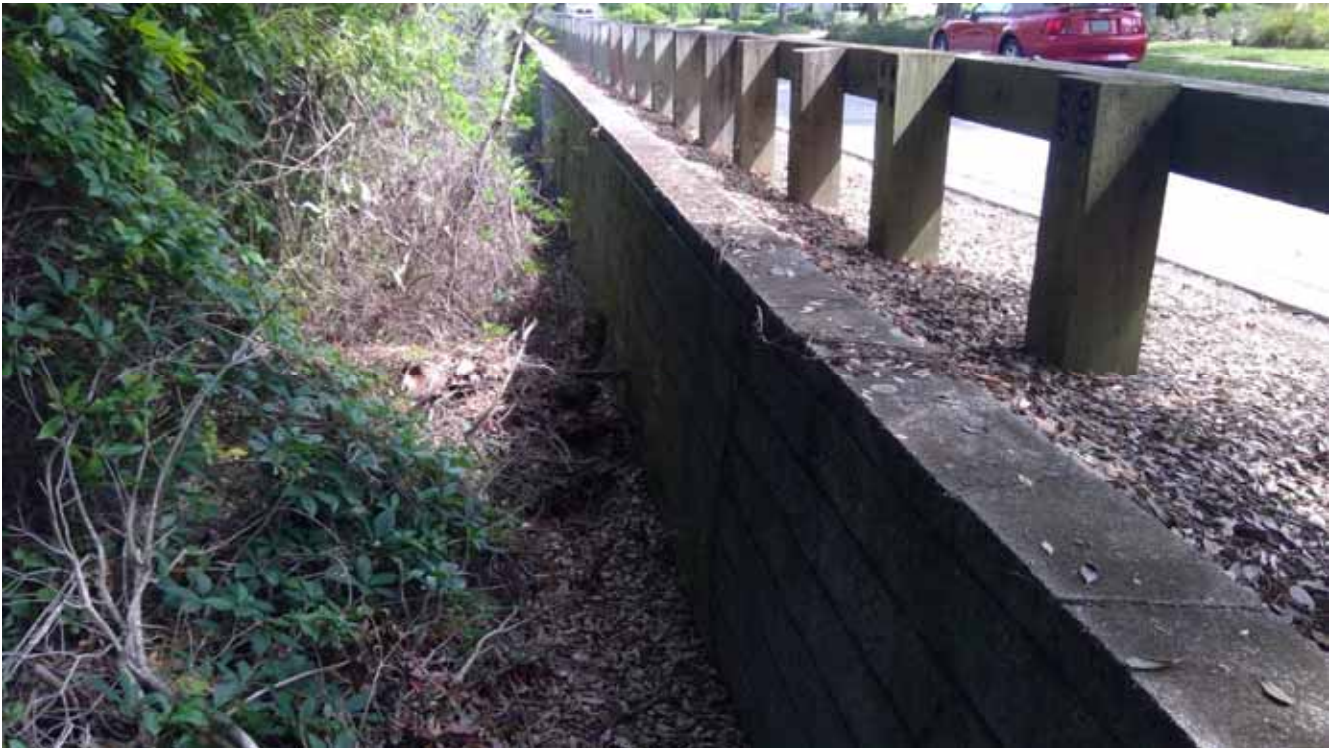
Retaining Wall - River Trail Dr
