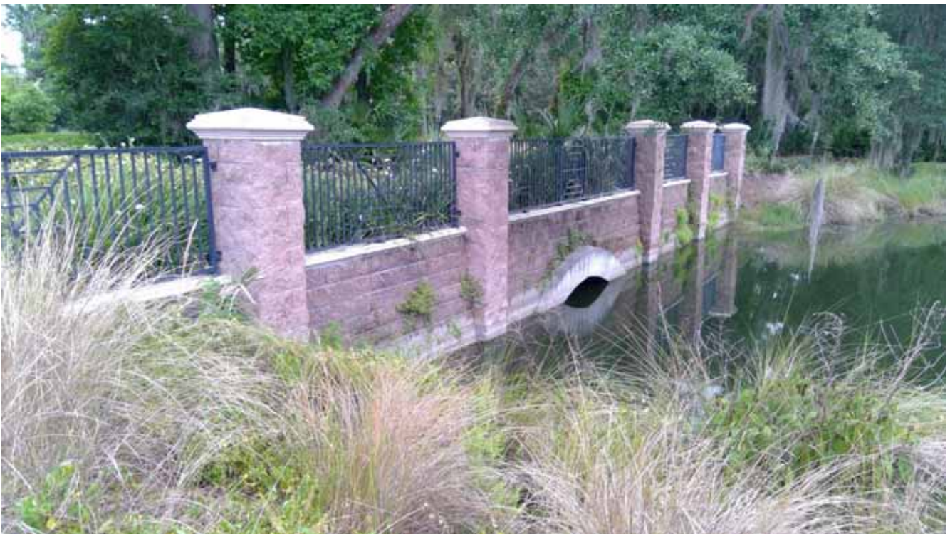
Culvert - Wild Oaks Entry
