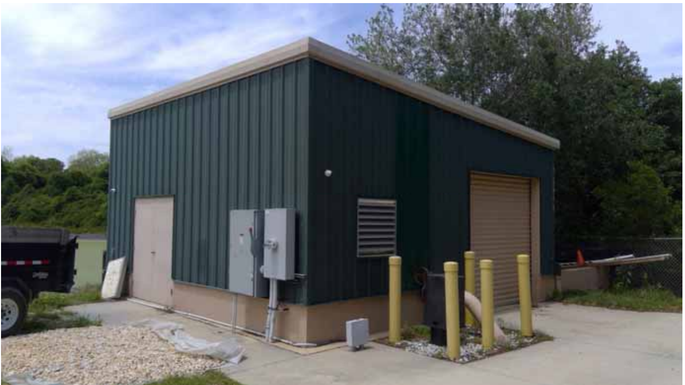
Pump House Building
