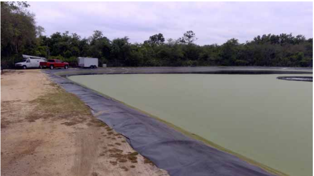
Irrigation Holding Pond
