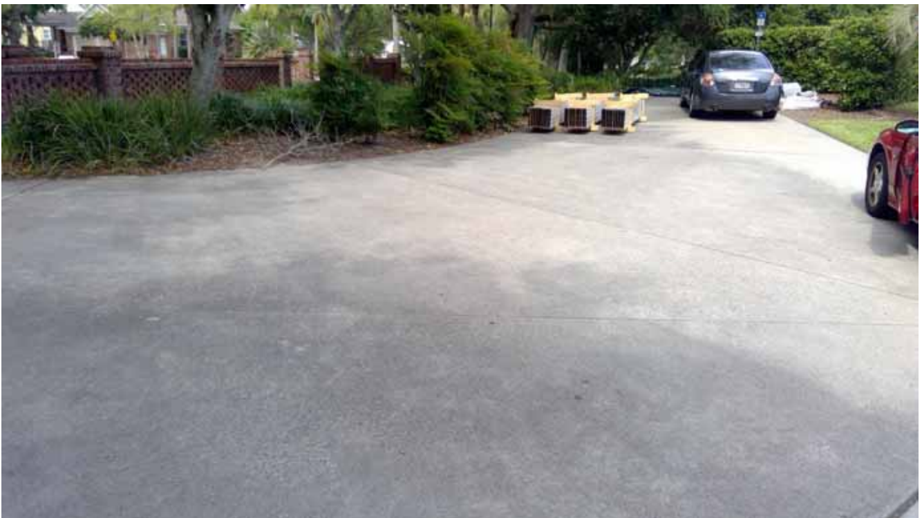
Parking Lot - Main Gatehouse
