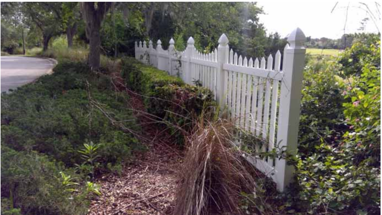
PVC Fence - Waterside Parkway
