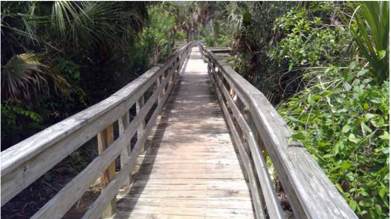
Boardwalk - Waterview Drive
