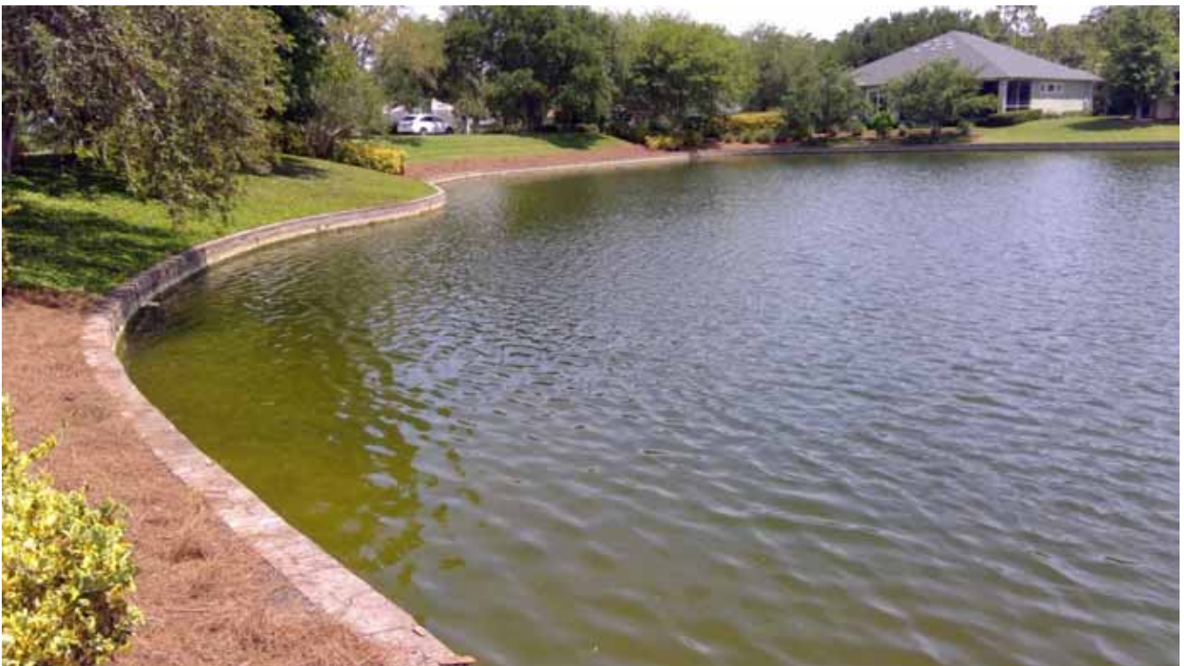
Bulkhead - Lake Haven
