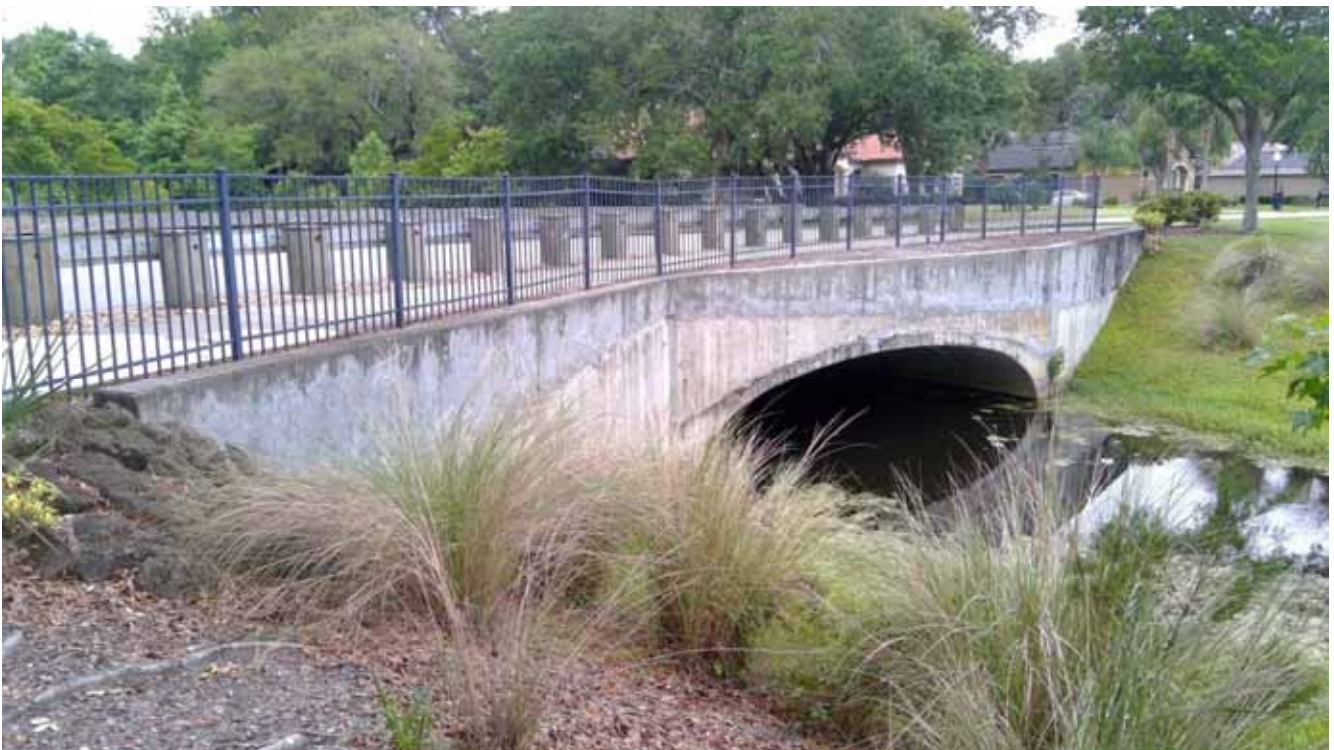
Bridge - WOW & Bluejack Ct
