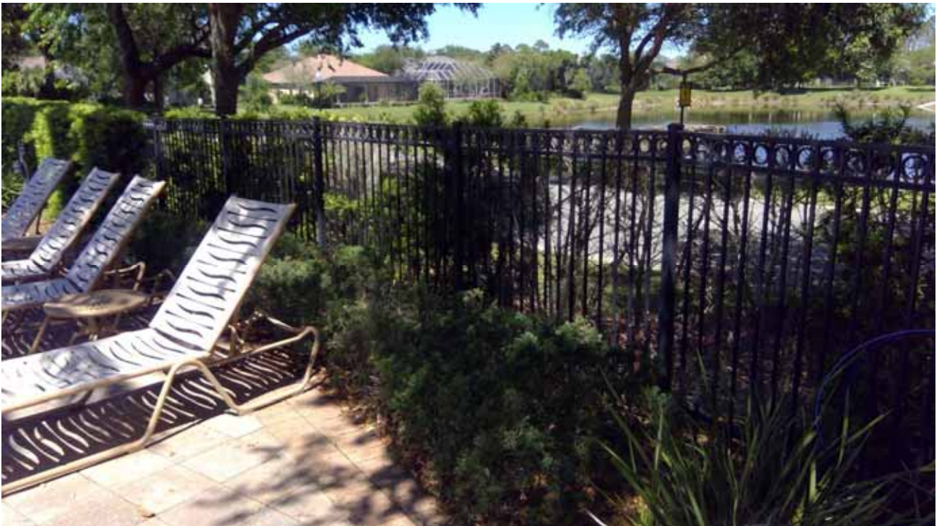
Fence - CAC Pool Deck
