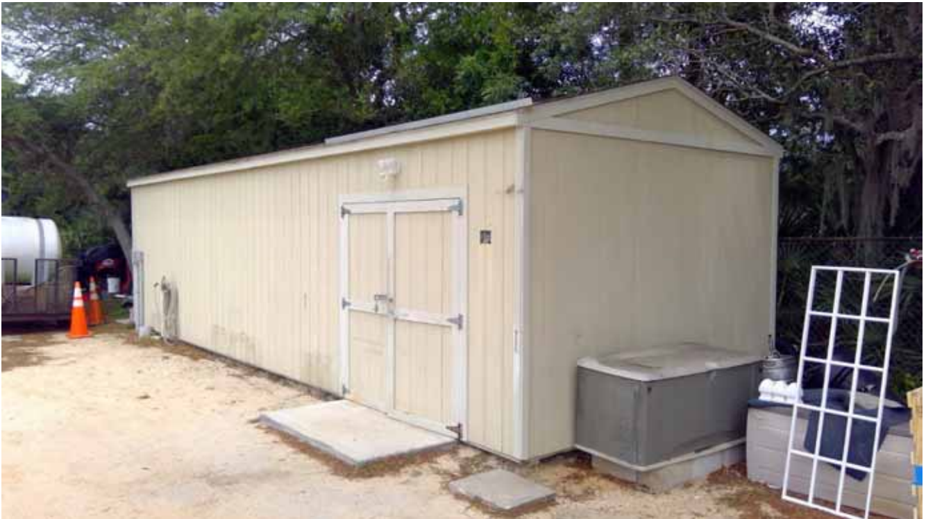
Storage Shed - Maintenance
